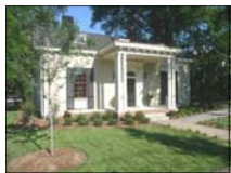
Bailey-Gallant House 507 N Blount St Closed & renovated. Legacy Construction offices.
