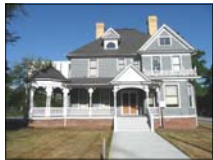
Jordan House 540 N Blount St Closed. Being renovated as offices for Holy Trinity Church.
