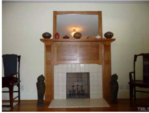
A custom crafted Arts and Craft style sawn-oak mantel surrounds the rebuilt fireplace. Master cabinetmaker Rhett Fulkerson also made the cabinets in the kitchen and bathrooms.
