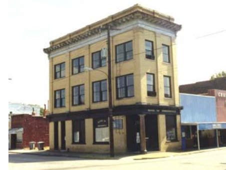
Bank of Robersonville, Robersonville, NC
