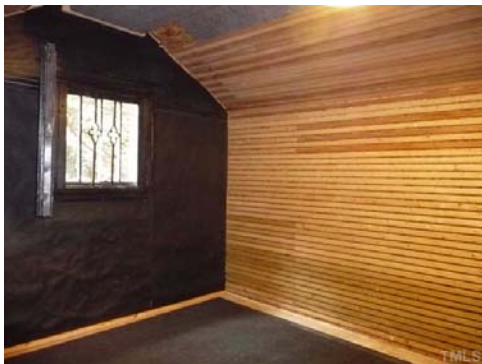
A separate exterior entrance behind the garage opens to a space used by a prior owner as an acoustically dampened drumming room and more recently by a tenant as potting studio.
